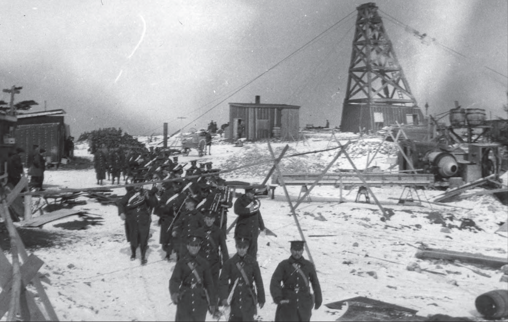
A military band leads a procession of troops to garrison Connaught Battery. The wooden tower (right) was part of the cable system used to lift loads up to the battery from the pier on the shore.
