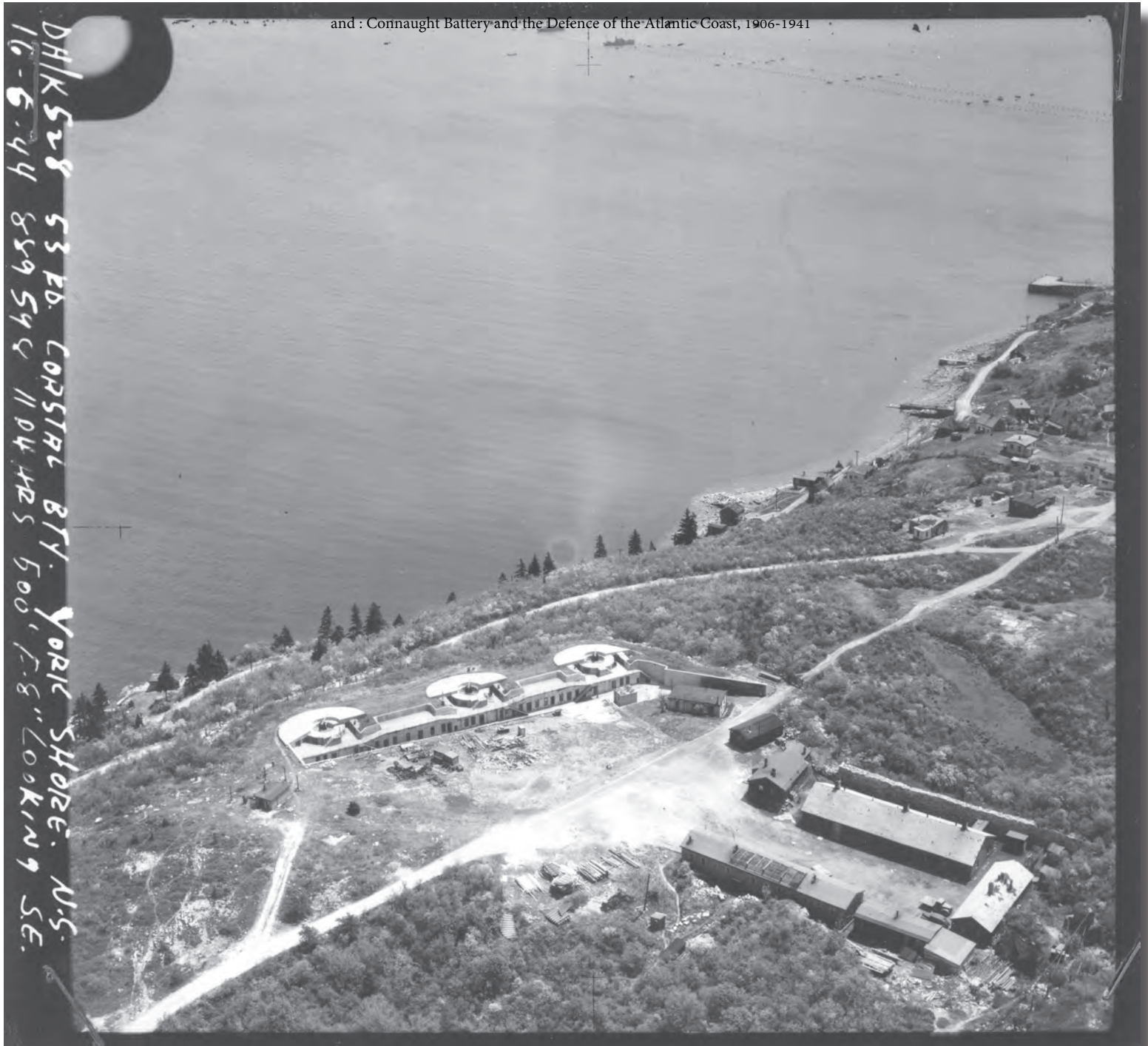
This air photo, taken in June 1944, shows Connaught Battery from the rear of the position. Note the anti-submarine nets in the top right corner of the photograph. By the Second World War the original guns had been replaced with dummy guns meant to deceive the enemy.
